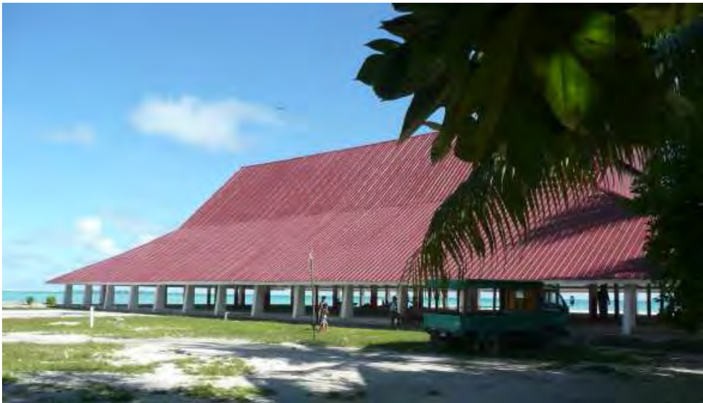
Figure 12 Very large maneaba at Teoraereke constructed in 2009 with no rainwater collection or storage.
