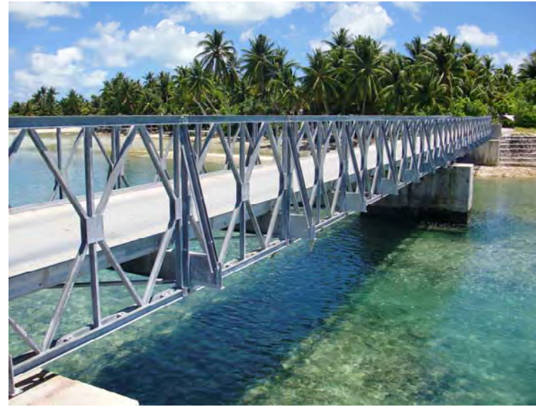
Photo No. 10 - The lower side rail is the recommended route from which the pipeline could be suspended.
