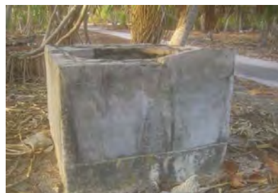
Fig. 2b-: Abandoned concrete water catchment
