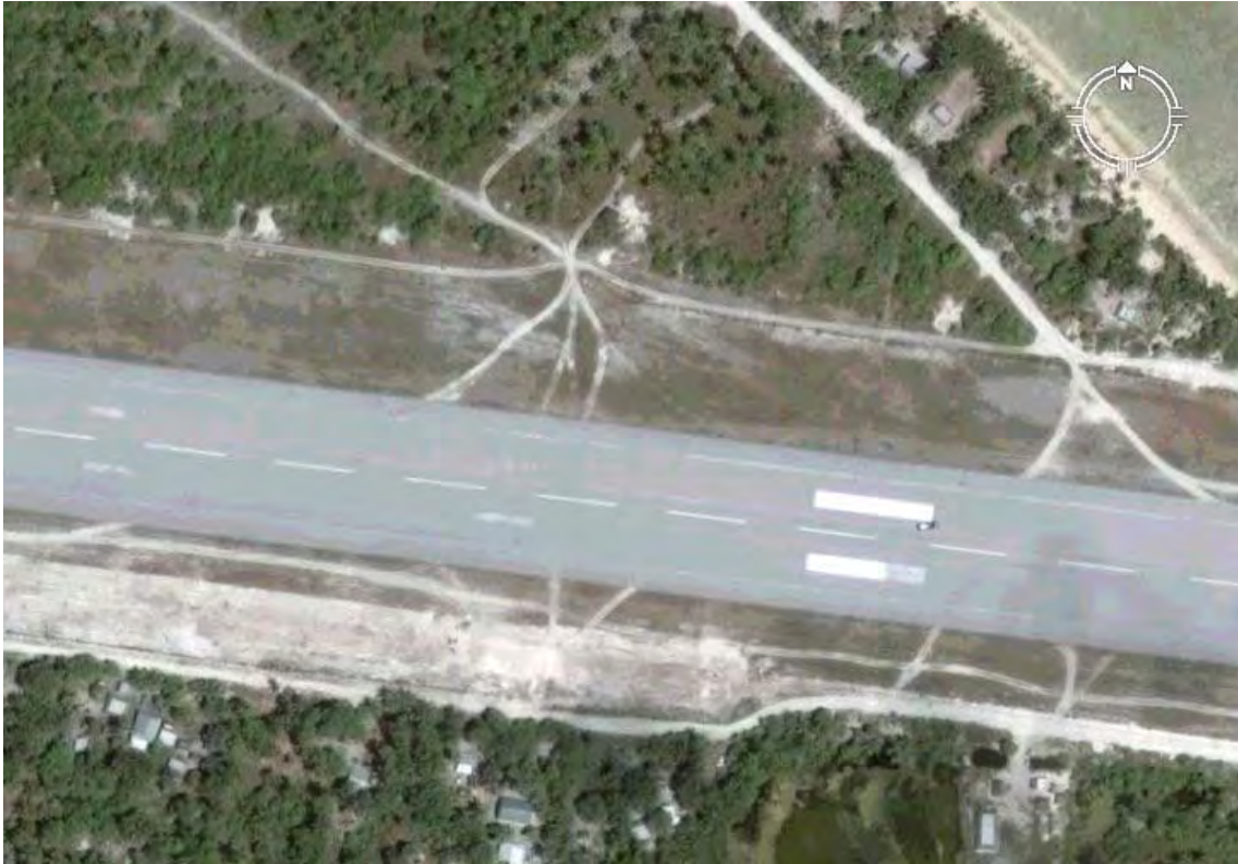
Figure 11. Sand and gravel mining within the Bonriki water reserve and close to gallery pump station PS1. The boundary road is again on the northeast ocean side (Google Earth).
