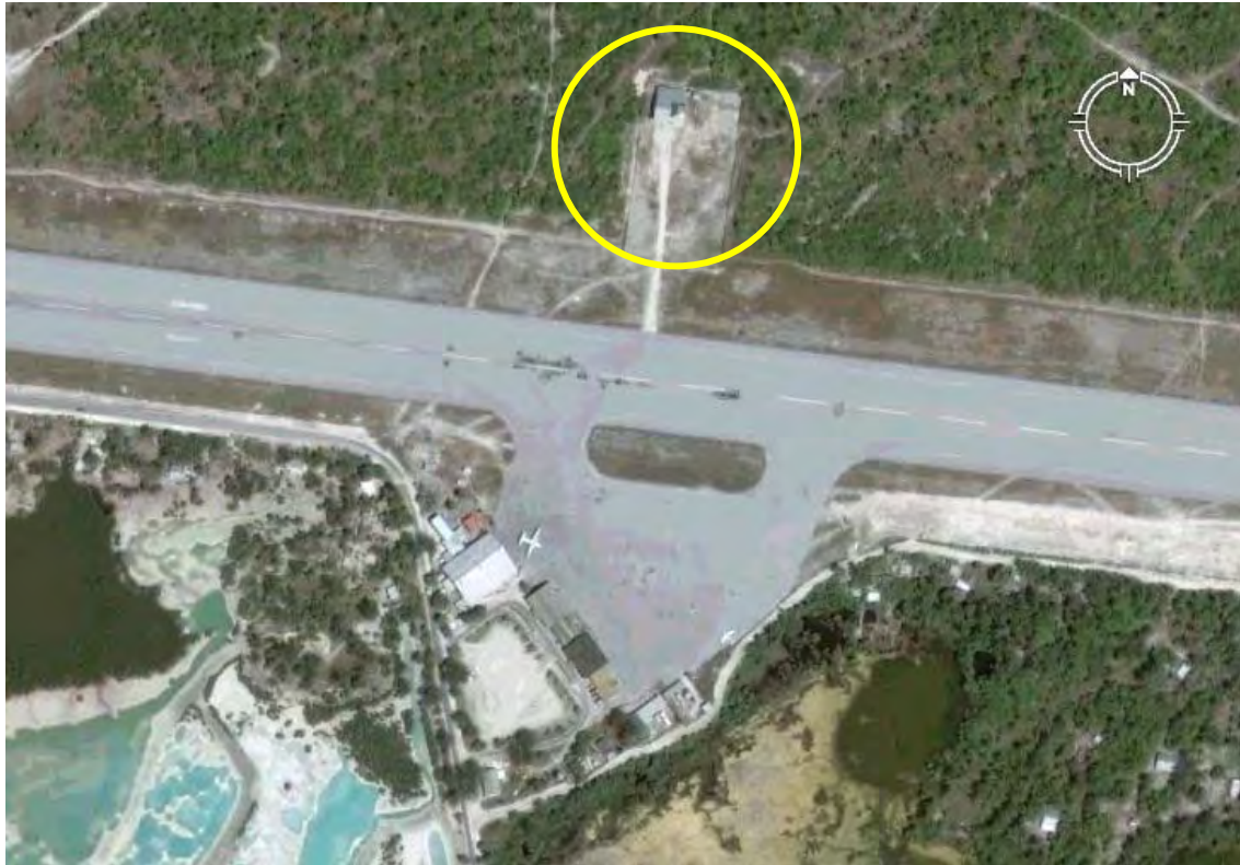
Figure 7. The Bonriki International Airport Control Tower (circled) located on the water reserve (Google Earth)
