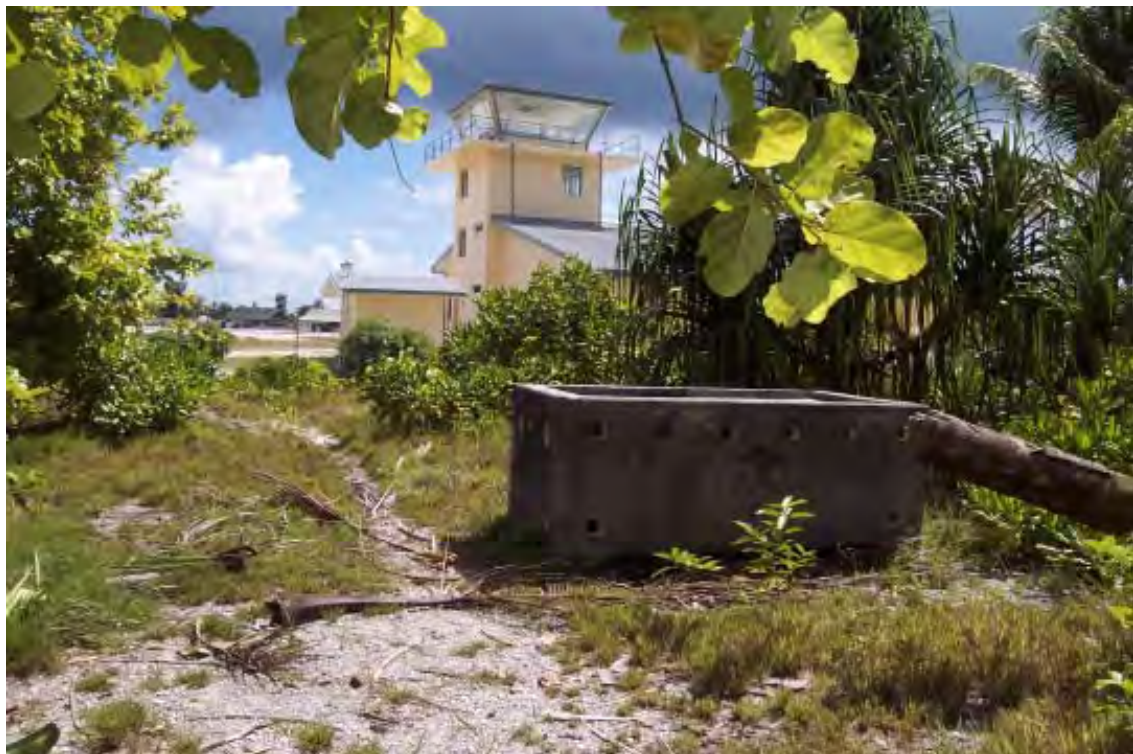
Figure 8. The septic tank toilet for the Control Tower is located over one of the infiltration gallery arms leading to Bonriki pump station 7 in the foreground right
