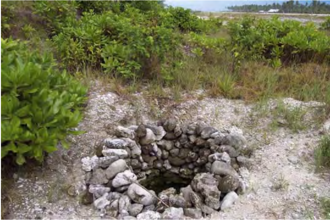
Figure 15. Open well dug down to the groundwater near PS 1. This has algal blooms growing on the water surface.
