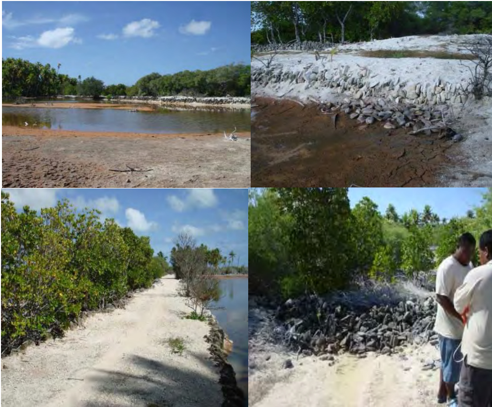
Fig. 2a: From top left to bottom right – coral boulder seawall; a closer look at the Tekarina seawall; a Taborara seawall almost turned into a causeway; the original strategy to reduce flooding and seawater intrusion (photos by Tion K.Uriam)
