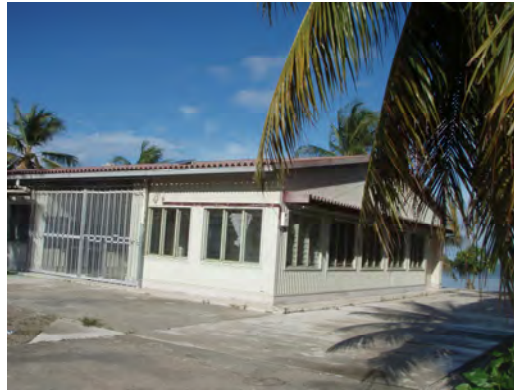
Fig. 2c: Kuria Ice Plant funded by JICA (photo by Erimeta Barako)
