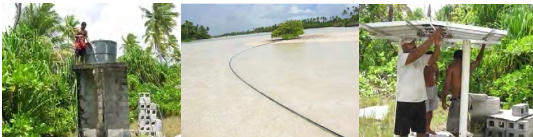
Fig. 2e: An overhead tank on an islet providing water for Anginbaiatooa Primary School, Keue; a pipe bringing water to the school; a solar pump (photo by Titeem Auatabu)
