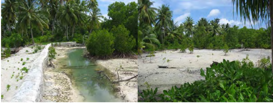
Fig. 2f: a concrete wall to reduce babai pit flooding; an eroded coastline giving way to flooding during extreme high tides (photos by Titeem Auatabu)
