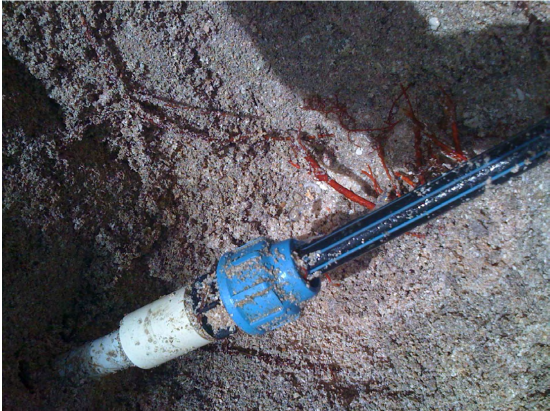
A “do it yourself” extension to get the water from the line closer to the house by forcing two pipe sections together. The only reason it didn’t blow apart was because of low system pressure. (See following photo)
